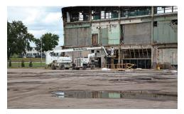
The outer structure of steel and masonry remained mostly intact but was under a great deal of stress. Brandenburg isolated the office structure from the fire-damaged areas. This allowed the customer an opportunity to determine the viability of reclamation of the remaining structure.
